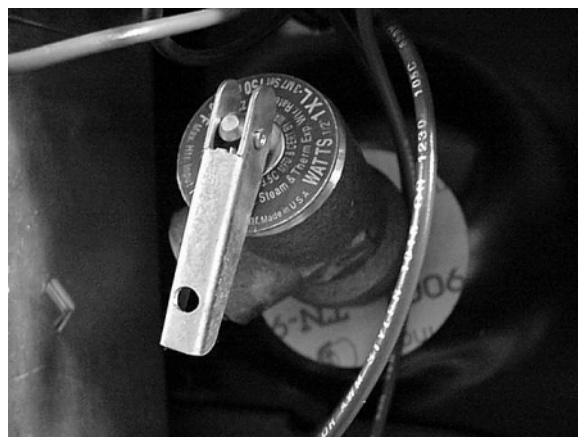
Lift straight out to open P-T valve
