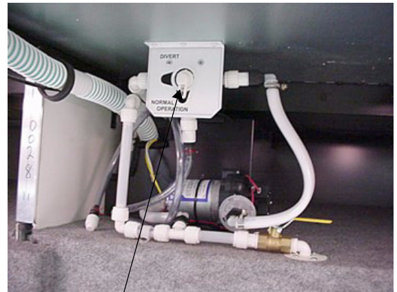
Water Heater By-Pass Valve
