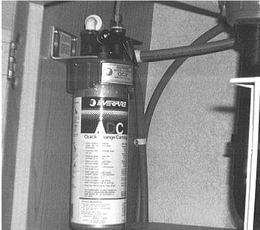
Water Filter Assembly - Below Galley Sink
