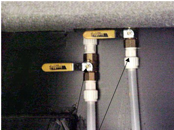
Water Line Drain Valves (in water center compartment)
