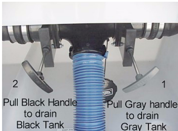
Holding Tank Valves (Typical)
