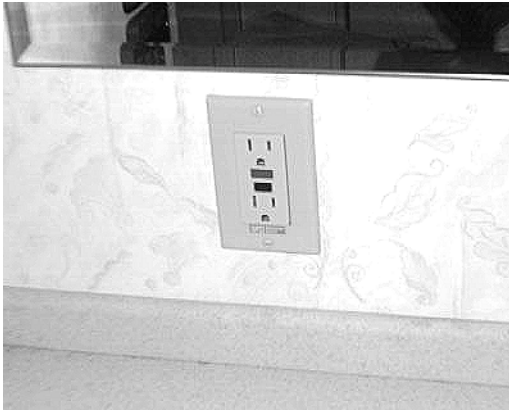
Ground Fault Circuit Interrupter (GFCI)
