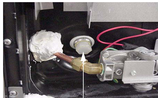
Water Heater Drain Plug (Remove with socket)
