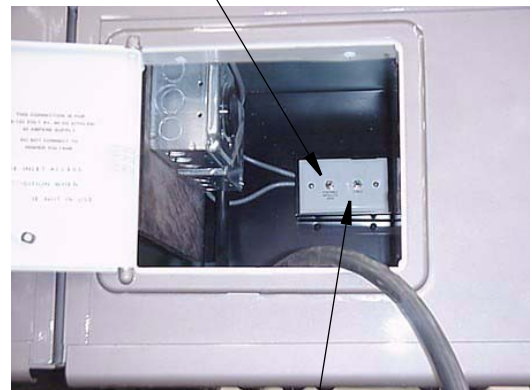
Portable Satellite Dish Hook-up in Shoreline Compartment
