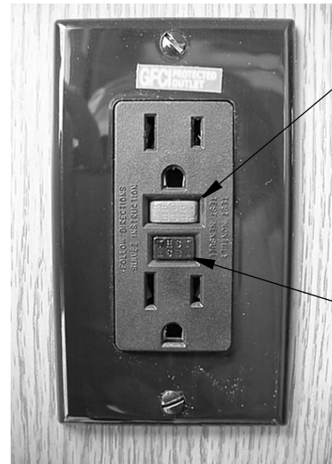
GFCI Outlet (Ground Fault Protector)
