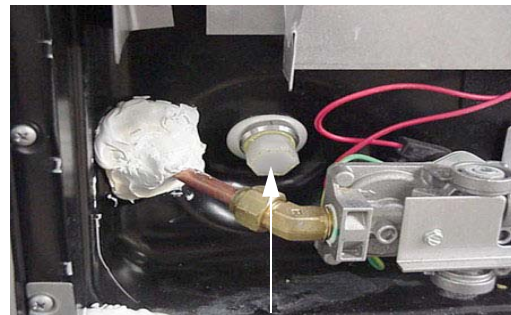
Water Heater Drain Plug (Remove with socket)
