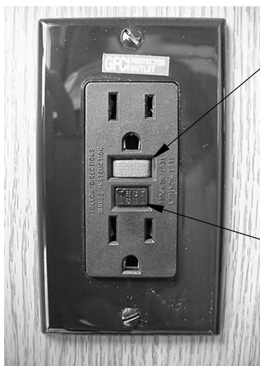
GFCI Outlet (Ground Fault Protector)
