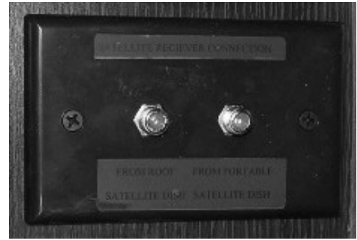
Interior Connection for Satellite Dishes Models 37F and 35Z only (Located in cabinet near TV) - Typical View
