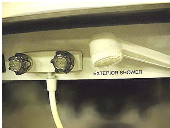
Exterior Shower/Wash Station -Typical View
