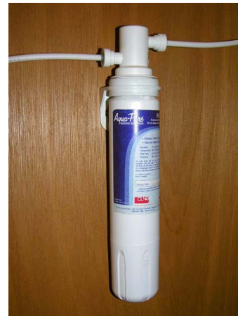
Water Filter Assembly below Galley Sink
