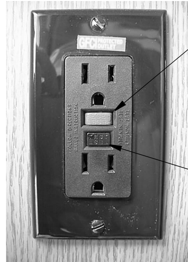
GFCI Outlet (Ground Fault Protector)
