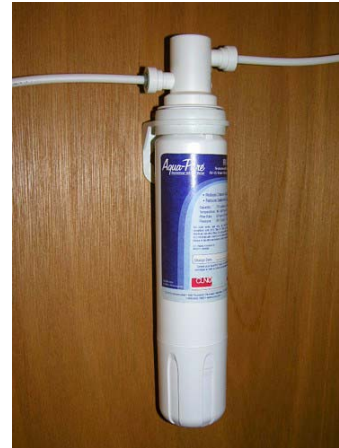
Water Filter Assembly (Located below Galley Sink)
