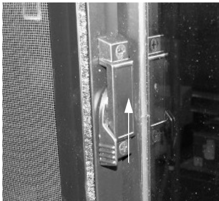
Pull latch UP to slide window open
