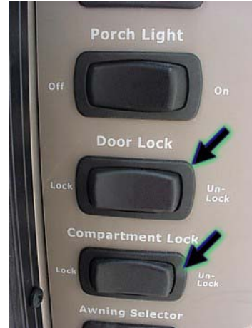
Power Door Locks (Located on entry switch panel) -Typical View
