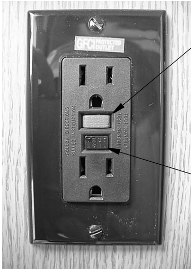
GFCI Outlet (Ground Fault Protector)
