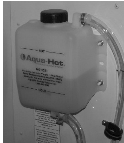
Expansion Fill Tank
