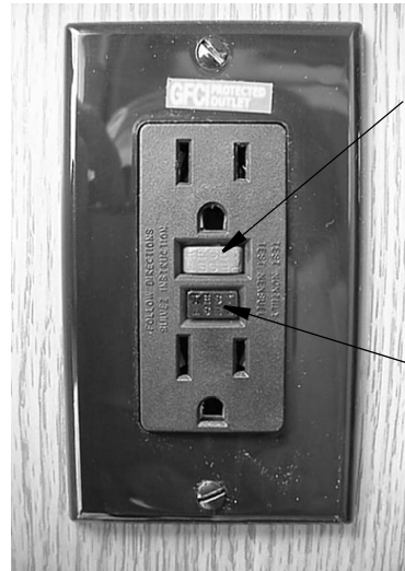
GFCI Outlet (Ground Fault Protector)
