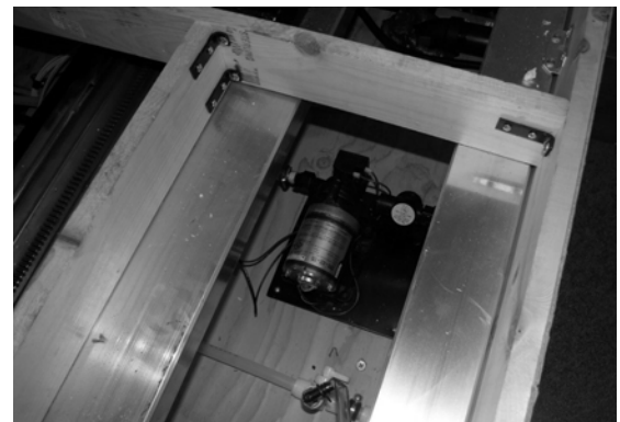
Water Pump (Located underneath bed) -Typical Installation
