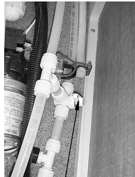
Waterline Drain Valve (Typical)
