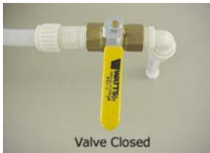
Water Tank Drain Valve (Typical)
