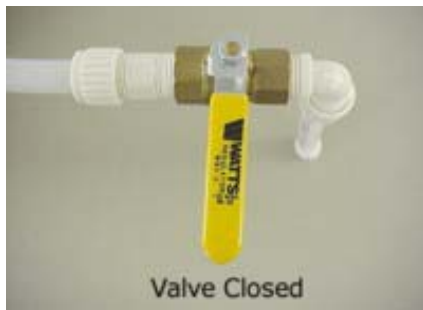
Water Tank Drain Valve (Typical)
