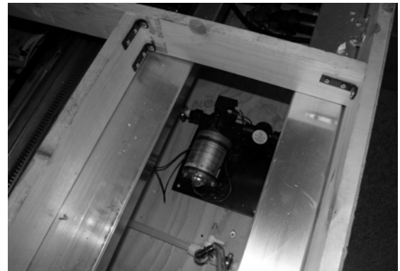
Water Pump (Located underneath bed) -Typical Installation
