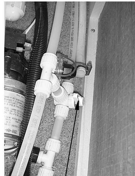
Waterline Drain Valve (Typical)
