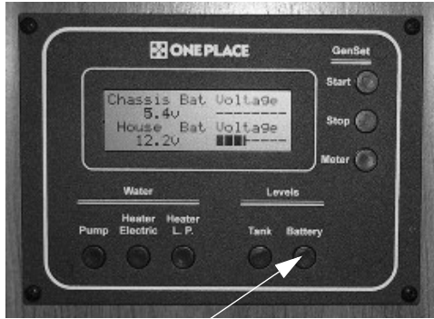
Battery Levels Switch
