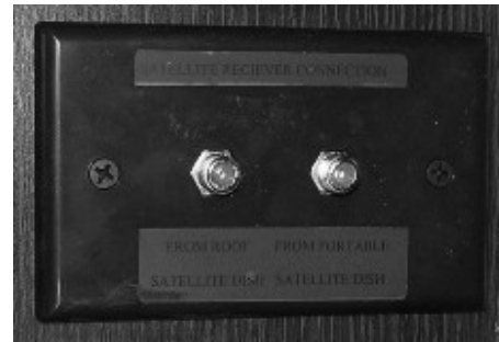
Interior Connection for Satellite Dishes (Located in cabinet or on a wall near TV) -Typical View
