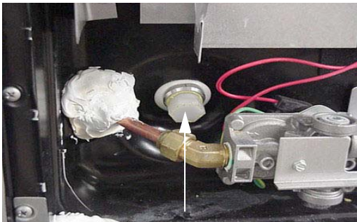
Water Heater Drain Plug (Remove with socket)
