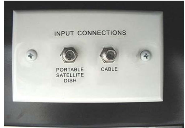
Satellite and Cable TV Hook-Ups (Located in shoreline or utility compartment - depending on model)
