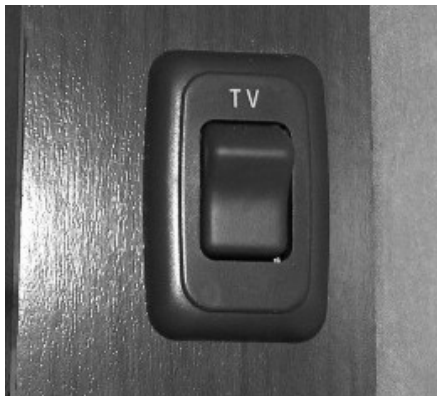
12V TV/DVD Master Power Switch (Located on cabinet or wall near TV) -Typical installation shown
