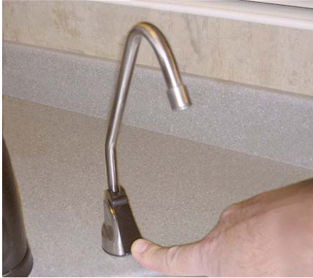
Filtered Water Faucet -Typical View
