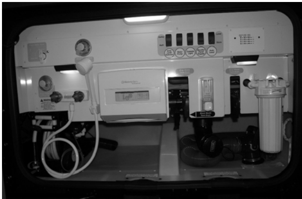
Water Service Center -Typical View
