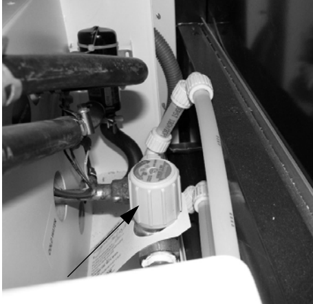
Hydronic Heating System Tempering Valve (Located on back side of the Aqua-Hot unit)
