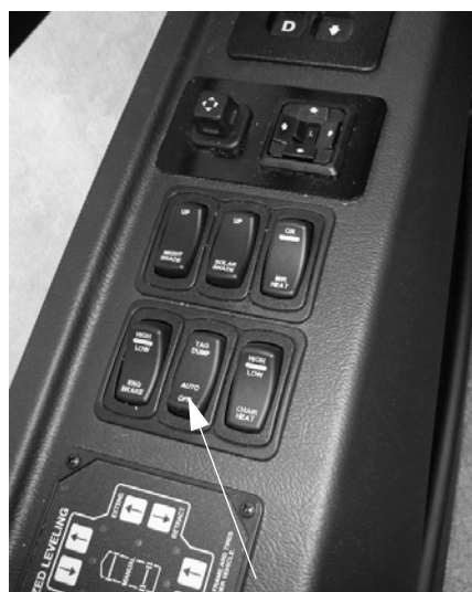
Tag Axle Switch (Located on the driver side trim panel) -Typical View
