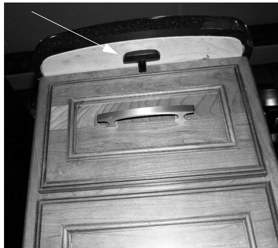
Countertop Extension Release Lever (Located underneath countertop extension lip) -Typical View
