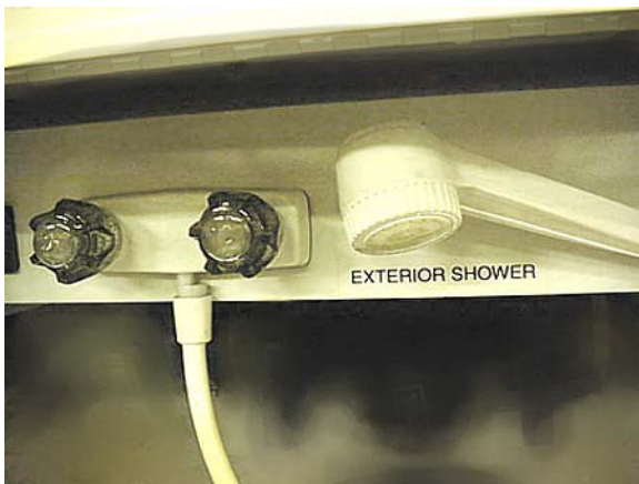
Exterior Shower/Wash Station -Typical View
