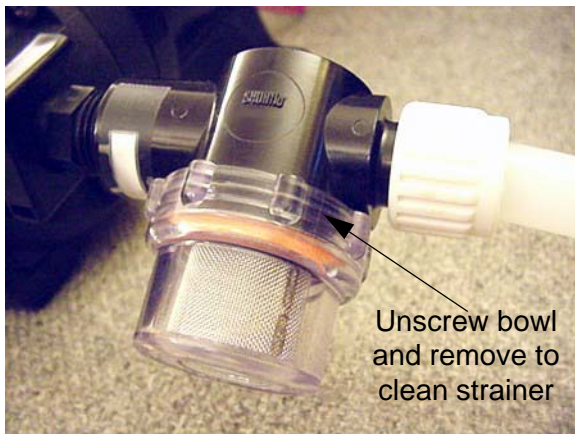
Water Pump Strainer -Typical View
