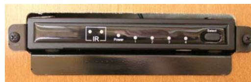
Secondary Source Selector (Located near each TV)
