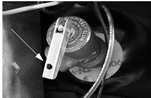
Pressure Temperature Relief Valve (Lift handle only when water heater is cold)
