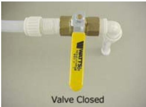
Water Tank Drain Valve (Located in water service center - pull to drain)
