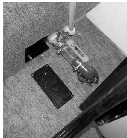
Water Tank Drain Valve (Located in first passenger side compartment)
