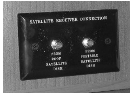
Interior Connection for Satellite Dishes (Located in cabinet or on a wall near TV) -Typical View
