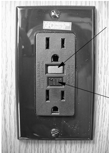
GFCI Outlet (Ground Fault Protector)
