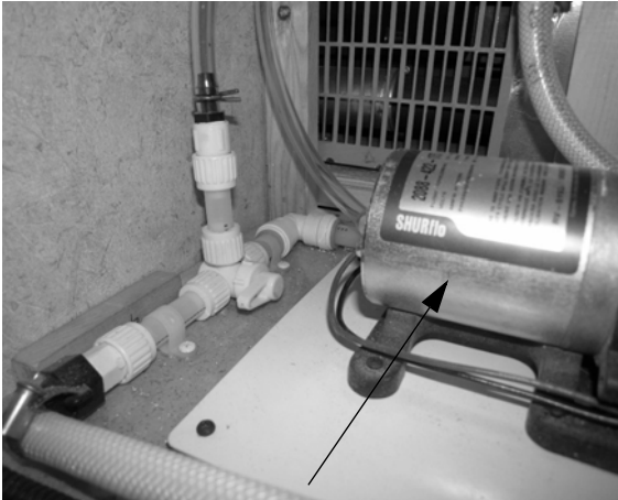
Water Pump -Typical installation shown
