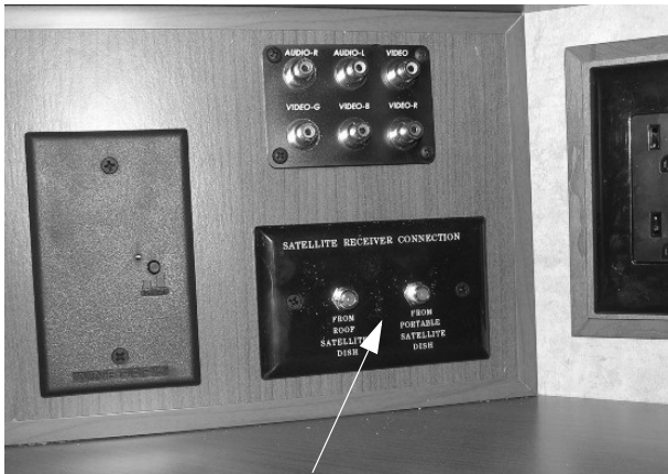
Interior Satellite Dish Connections (Located in galley or bedroom overhead cabinet) -Typical installation shown
