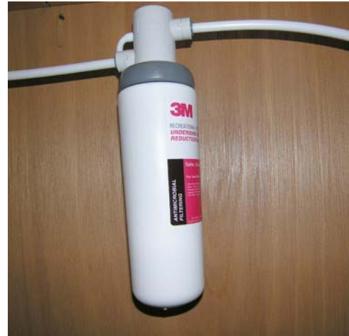
Cold Water Filter Assembly (Located below galley sink) NOTE: Hot waterline is not filtered
