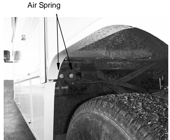
Rear Air Spring Valves (Located inside left rear wheel well -Typical View
