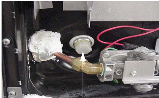
Water Heater Drain Plug (Remove with socket)
