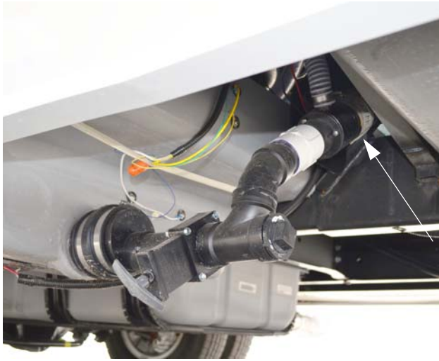
Waste Pump (Located on driver side of coach behind rear wheel) -Typical View
