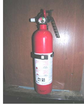
Fire Extinguisher (Typical installation - your coach may vary according to model and floorplan)
