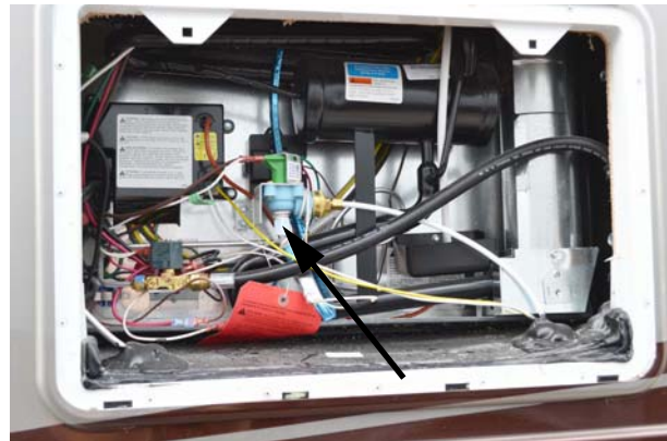
Ice Maker Water Supply Connection -Typical View
