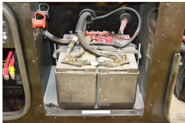
Chassis Batteries -Typical View
