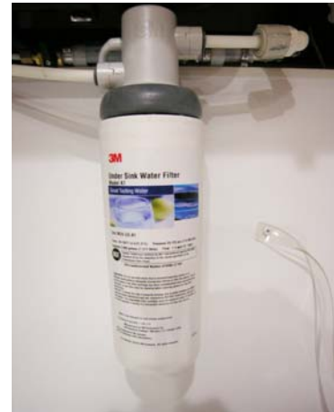
Filtered Cold Water/ Ice Maker Filter (Located below galley sink)
