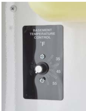
Basement Temperature Control
