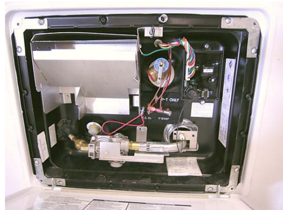
Water Heater Exterior Service Access -Typical View
