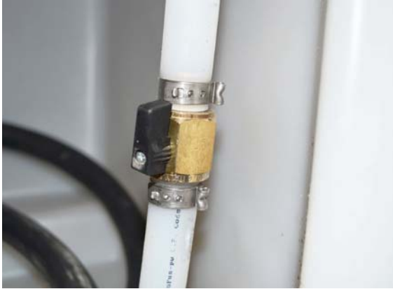
Water Tank Drain Valve -Typical installation shown
