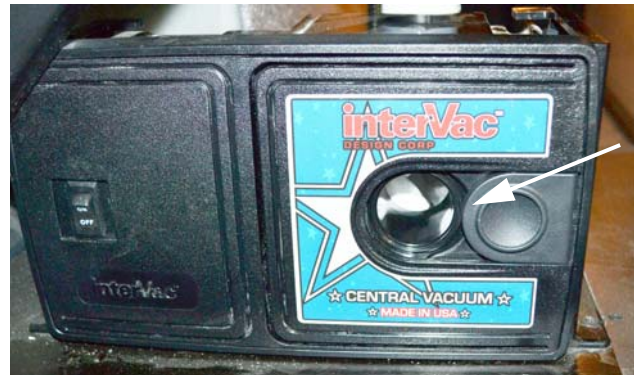
Exterior Hose Outlet
