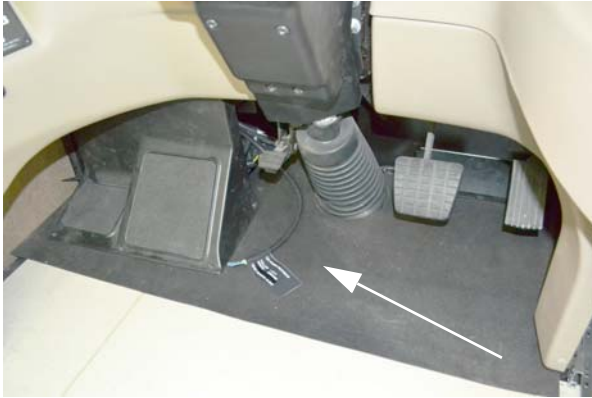
CB Power Wires -Typical View
