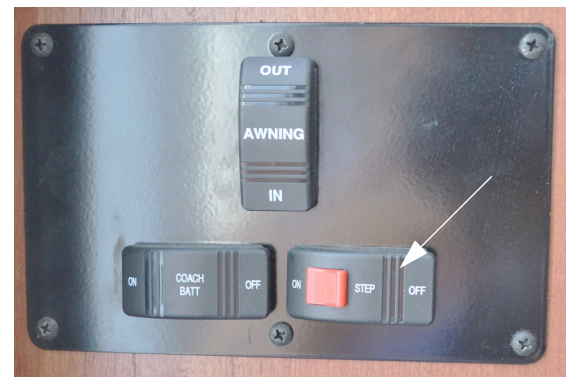
Entry Step Switch (Located near entrance door) -Typical View
