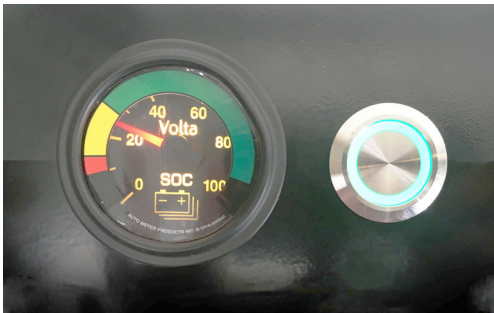
Pure 3 State of Charge (SOC) Gauge (Located on an interior cabinet) -Typical View
