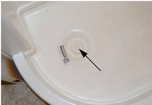
Shower Drain Strainer (Located in shower floor) -Typical View
