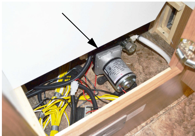
Shower Pump (Located beneath galley cabinet access panel) -Typical View
