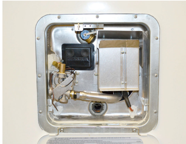
Water Heater Exterior Service Access
