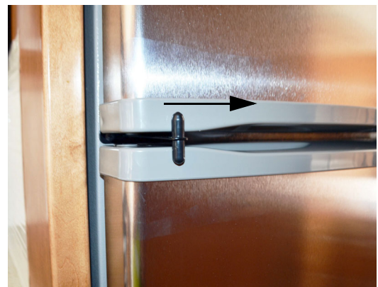
(Latch shown in lock position) -Typical View
