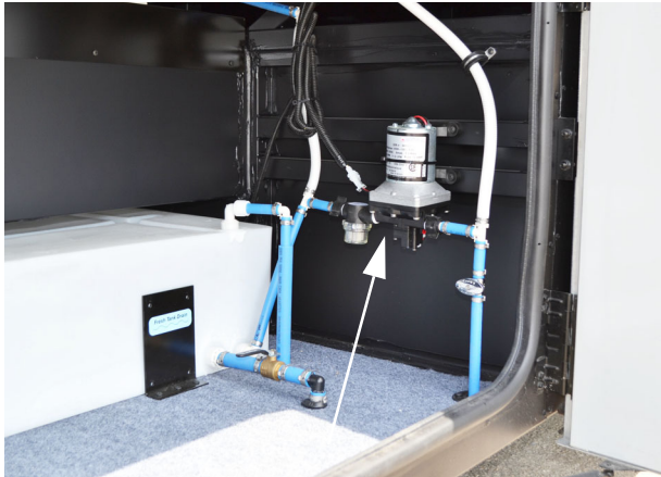
Water Pump (Located in a passenger side compartment) *Model 36G
