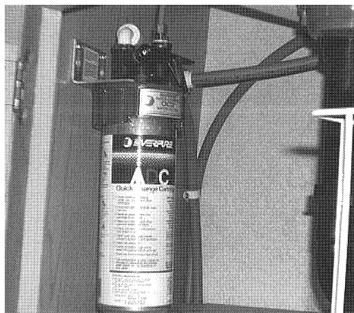
Water Filter Assembly - Below Galley Sink
