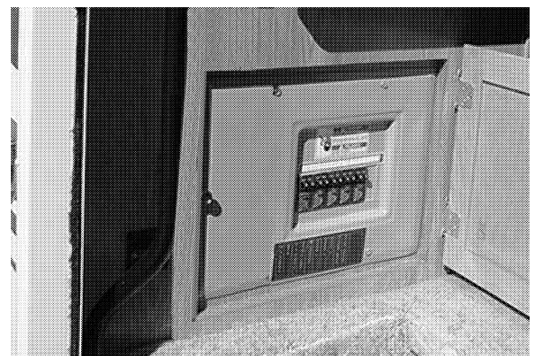
110-Volt Circuit Breaker Panel (Basement Models)
