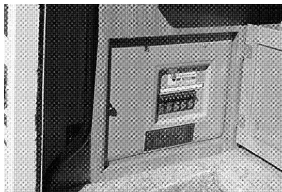
110-Volt Load Center - Basement Models
