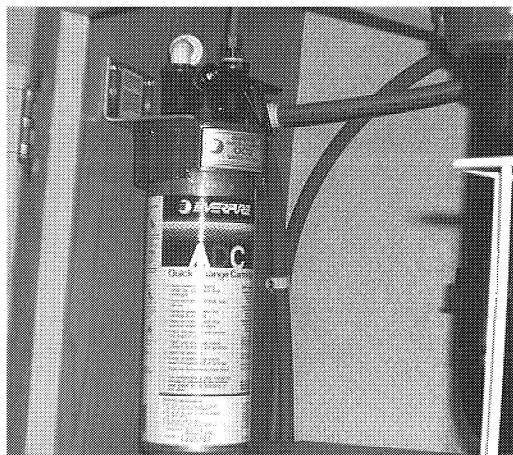
Water Filter Assembly - Below Galley Sink
