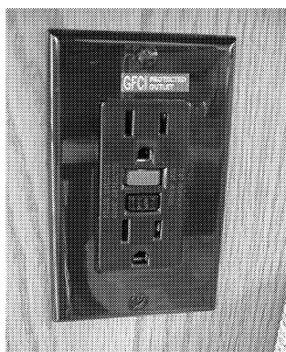
GFCI Outlet (Ground Fault Protector)
