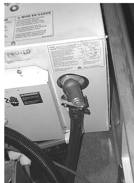
Pressure-Temperature Relief (P-T) Valve
