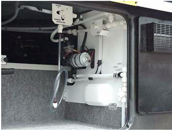
Water Pump and Filter in Right Front Shower Compartment
