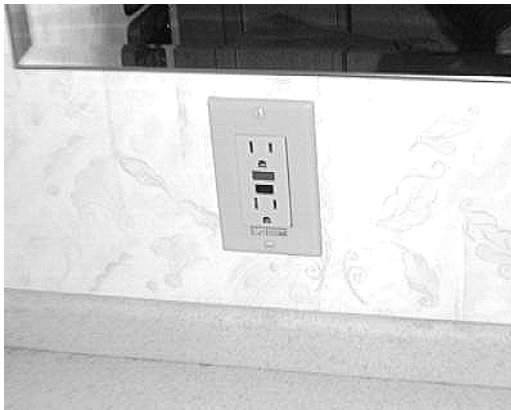
Ground Fault Circuit Interrupter (GFCI)
