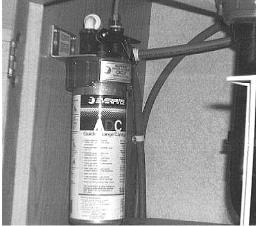
Water Filter Assembly - Below Galley Sink
