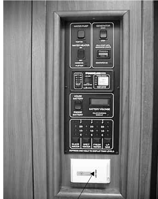
Power Vent Thermostat Bath Area
