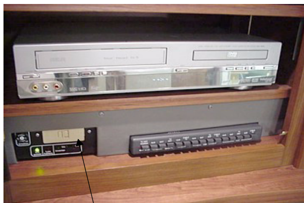
DC-AC Voltage Inverter in Video Center
