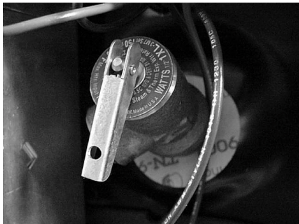
Lift straight out to open P-T valve
