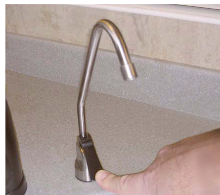
Filtered Water Faucet
