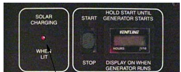
Solar Charging Indicator
