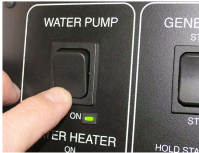
Water Pump Switch
