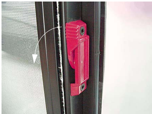
Pull latch outward to slide window open
