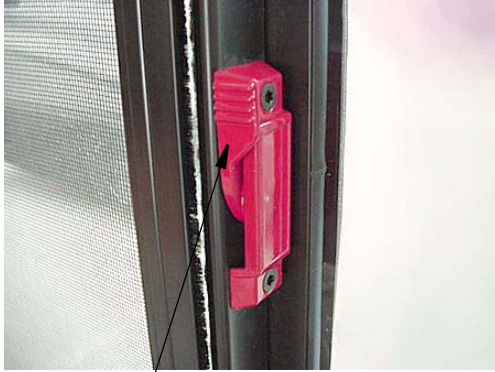
Pull latch outward to slide window open
