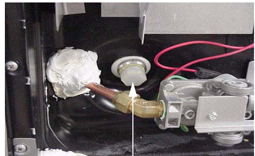
Water Heater Drain Plug (Remove with socket)
