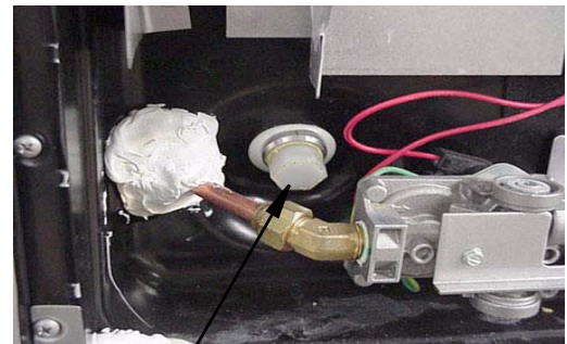
Water Heater Drain Plug Remove with socket
