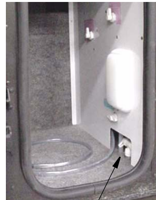
Water Line Drain Valve
