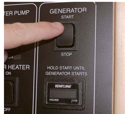
Generator Switch and Hourmeter
