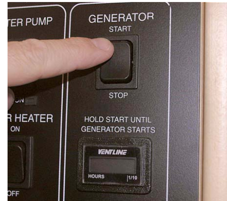
Generator Switch and Hourmeter on monitor panel
