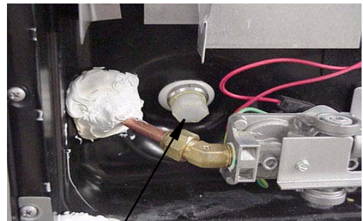
Water Heater Drain Plug Remove with socket
