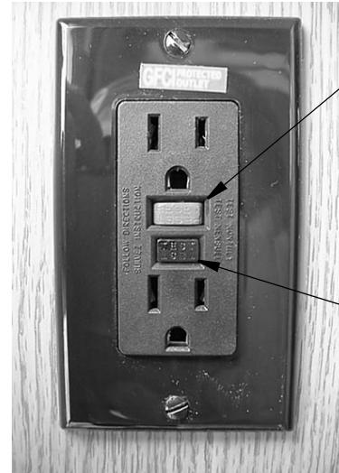
GFCI Outlet (Ground Fault Protector)
