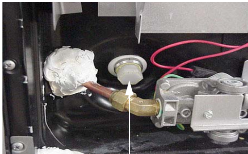
Water Heater Drain Plug (Remove with socket)
