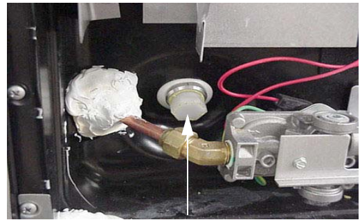
Water Heater Drain Plug (Remove with socket)
