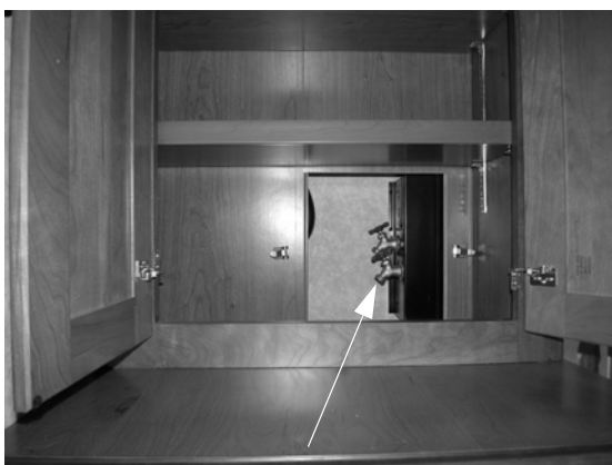
Water Supply Faucets -Typical Installation
