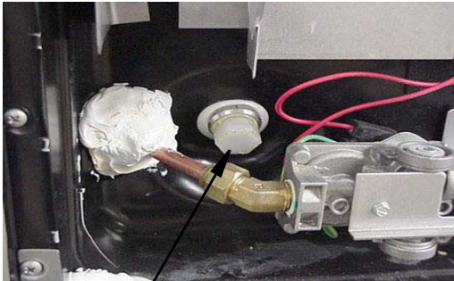
Water Heater Drain Plug (Remove with socket)
