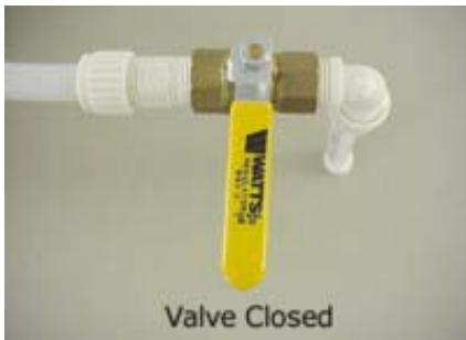
Water Tank Drain Valve -Typical installation shown
