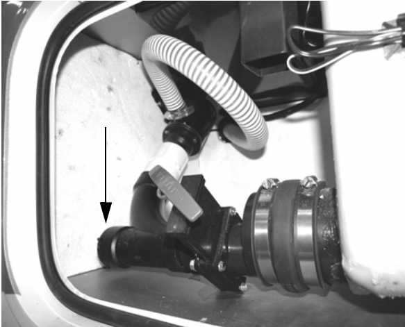
Waste Pump Drain (Located in driver side compartment behind rear wheel)
