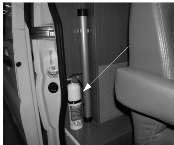
Fire Extinguisher (Located near sliding entrance door) -Typical installation shown
