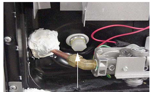
Water Heater Drain Plug (Remove with socket)
