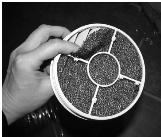
Air Filter (Located on back side of Return Air Vent) -Typical View
