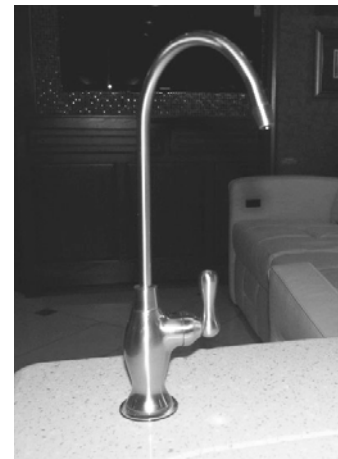
Filtered Water Faucet -Typical View
