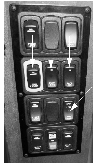
Awning Control Switches (Located near entrance door) -Typical View
