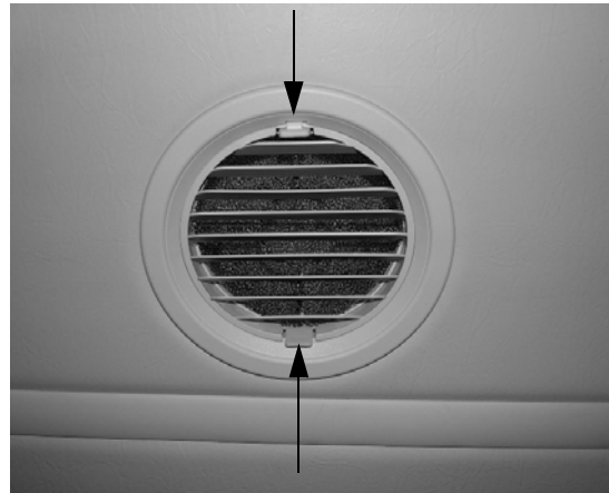
Return Air Vent (Press tabs inward to remove air vent) -Typical View
