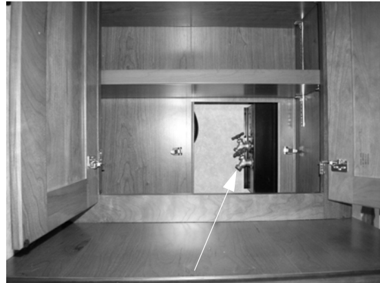
Water Supply Faucets -Typical installation shown
