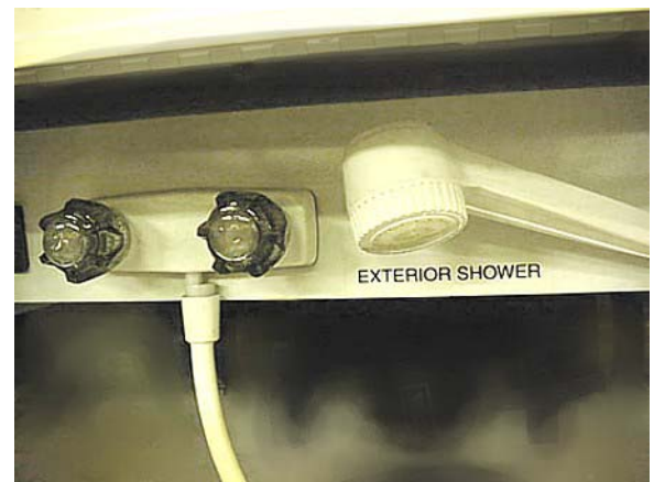
Exterior Shower/Wash Station -Typical View
