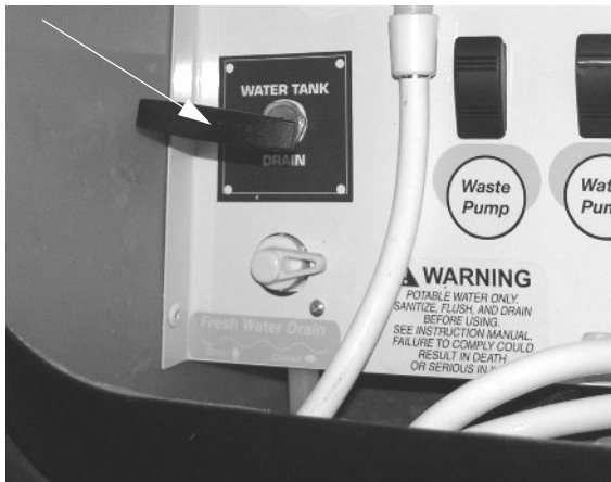
Water Tank Drain Valve -Typical installation shown
