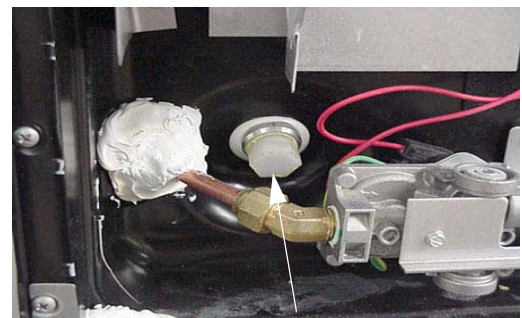
Water Heater Drain Plug (Remove with socket)
