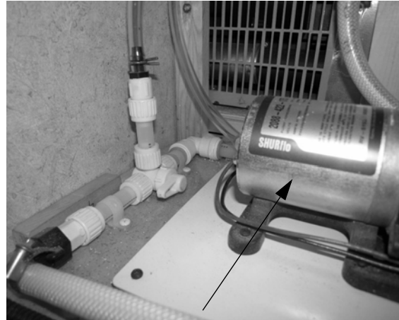
Water Pump -Typical installation shown
