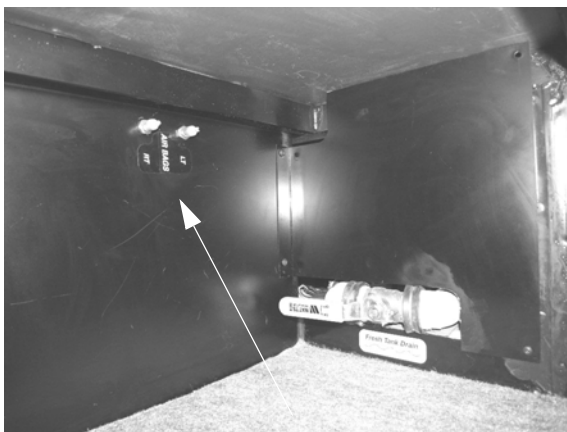
Rear Air Spring Valves (Located in rear driver side compartment)
