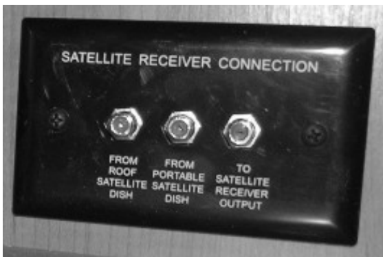
Interior Connection for Satellite Dish (Located near entertainment center cabinet) -Typical View
