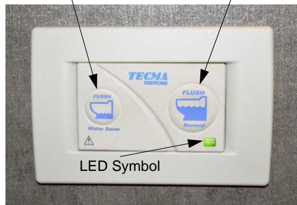
Wall Switch/Controller (Located on wall near toilet)
