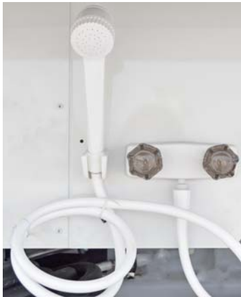
Exterior Shower/Wash Station -Typical View
