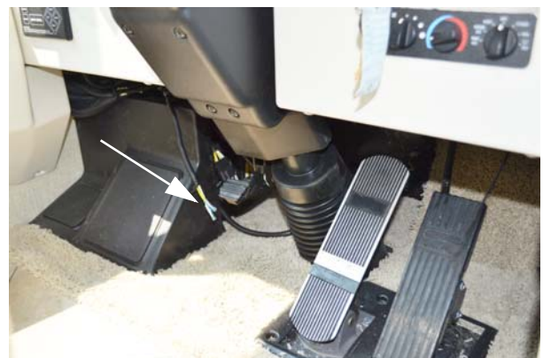
CB Power Wires -Typical View
